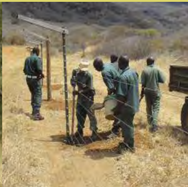
Rhino Sanctuary fence repair team at work
